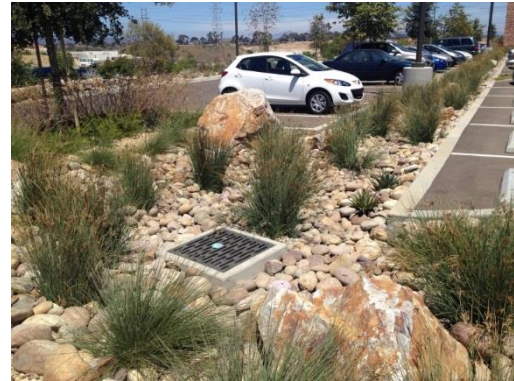
Figure 3-22. Biofiltration in a Parking Lot
