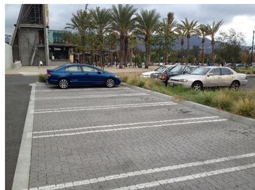
Figure 3-20. Bioretention and Permeable Pavement at the Los Angeles Zoological Park
